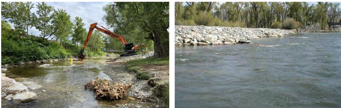
Fig. 2: Left: Instream River Training at the Brigach (Source: wald-corbe.de). Right: River Bank protection with riprap (Source: Trout headwaters, Inc).
